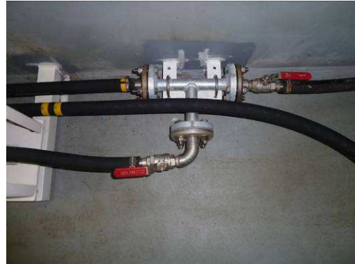
T connection, left to TSG - right to CO 2
