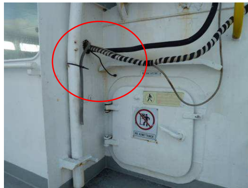
Bridge deck – top of the elevator
